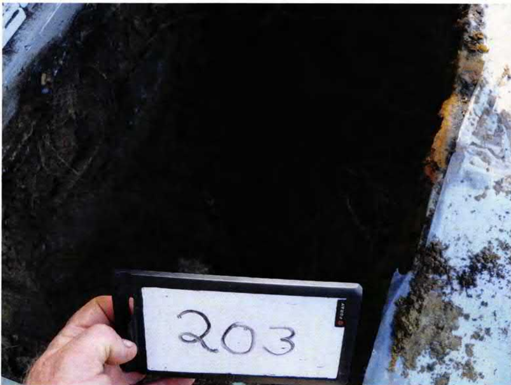
Picture 2: UST 203Balsam excavation.
